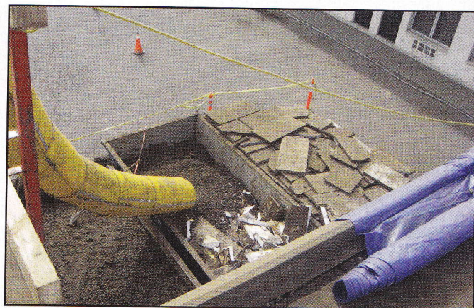
CRS had a subcontractor dry vacuum the existing roof gravel and debris. "They had to come off the main street and took up the whole lane with the giant vacuum truck and dump bin," says Justice.
