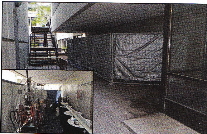
Where's the spray equipment? The CRS crew had it neatly obscured by this temporary wall. Shielding the equipment protects it from the elements and makes for a more organized spray foam application.
