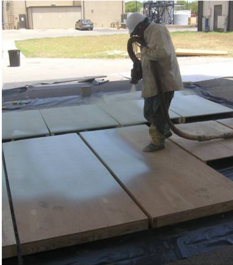
Figure B-1. Application of SPF.
